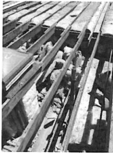
Attic Insulation in piles
