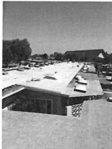
Plywood Sheathing 1 Bedroom
