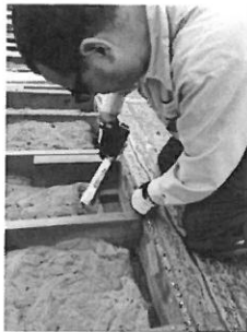
New Attic Vent Screens
