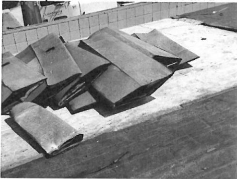
Remove square duct Replace with 7 inch round
