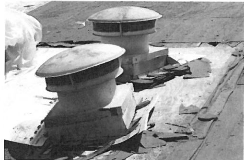
Remove Range Hood Fans from Roof
