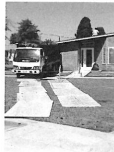
Roof debris drop and asset protection
